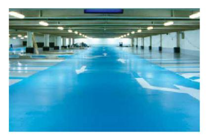
Enclosed, intermediate and lower decks and bays are protected from weather conditions to a large degree, and are less susceptible to stress than top decks, although still exposed to aggressive water born salts. Master Builders Solutions systems for light to medium duty operations take this into account with specific systems that are fit for purpose.
